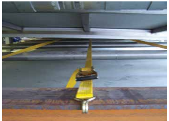
Example of Temporary Return Support
