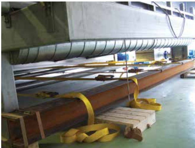
Example of Temporary Return Support
